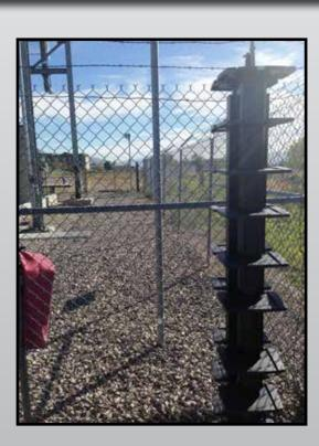
Active IR Signal between beams
