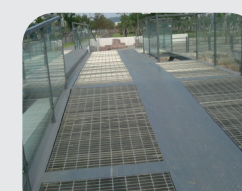
Steel grating and duckboards
